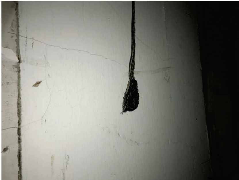
Photo 11: HA11 Black wall glue lines on the walls of the 2 nd floor classrooms (B31-B33) 3% Chrysotile
