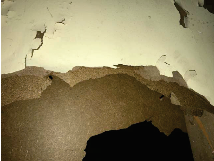
Photo 7: HA7 Brown felt paper in the walls in the 1 st floor hallway (B19-B21)
