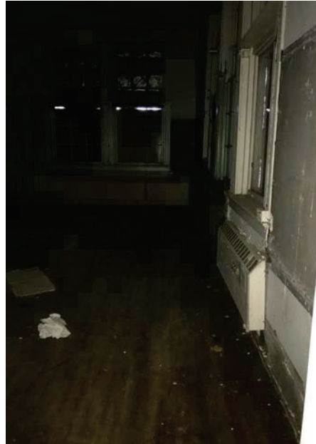
Photo 12: Classroom [1 st Floor, 1 st room on left]
