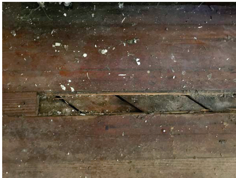
Photo 22: Closeup of Planking under Flooring
