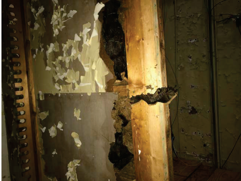
Photo 21: HA21 Brown insulation in the walls of the 1 st floor hallway (B59-B61)
