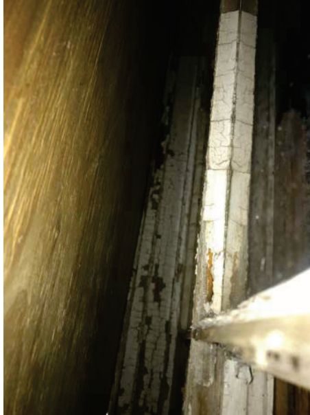
Photo 6: HA6 Exterior window glazing on the multiple panel windows throughout the subject property (B16-B18)
