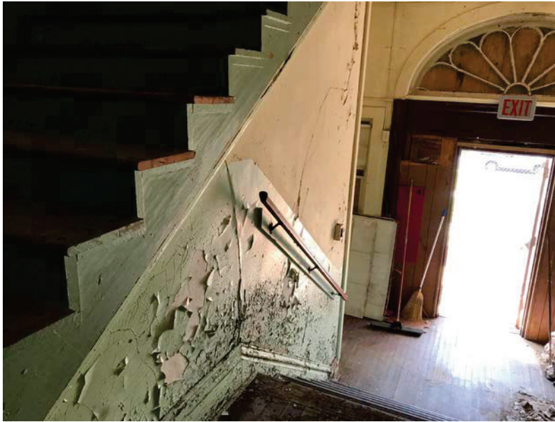
Photo 9: Entryway/Front Door [Looking towards Southeast]
