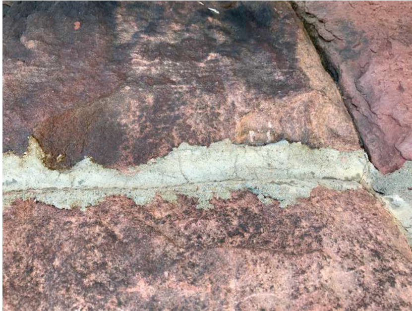
Photo 25: HA25 Gray brick mortar on the exterior of the subject property (B71-B73)
