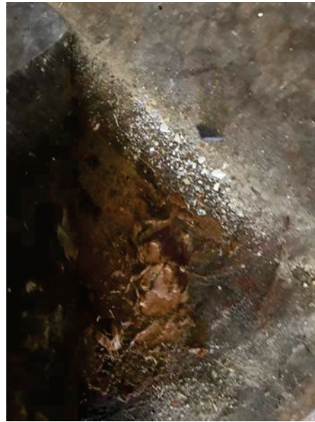
Photo 18: HA18 Brown stair covering and associated tan mastic on the stairwells of the subject property (B50-B52)
