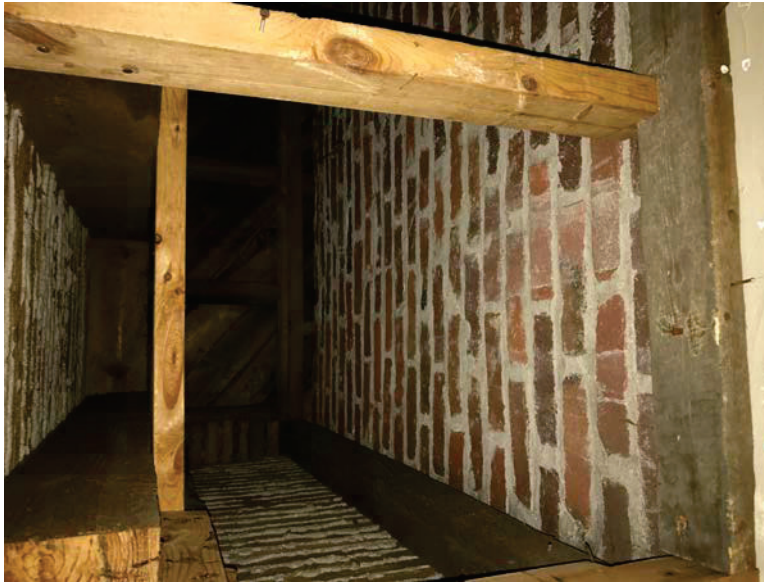
Photo 21: Planking under Hardwood Flooring
