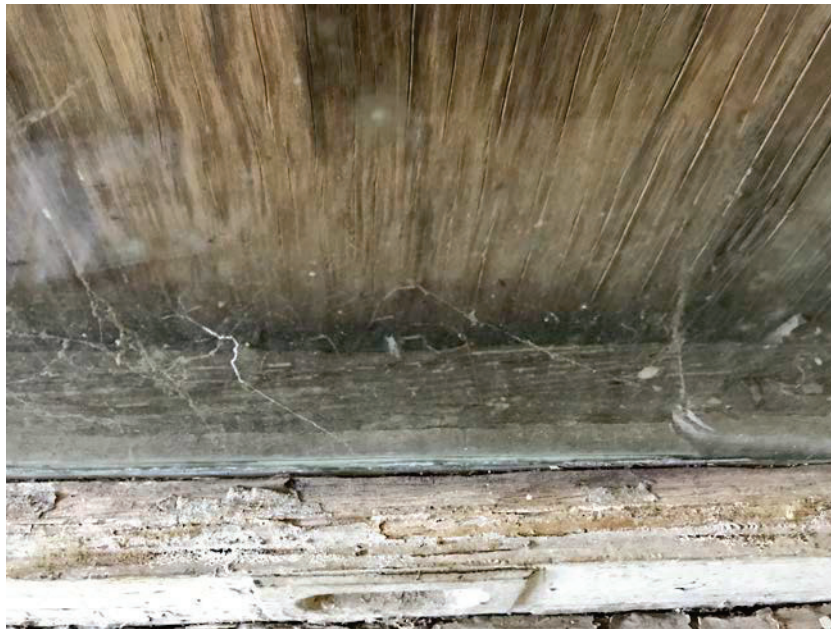
Photo 20: HA20 Exterior window caulking on the single panel windows of the subject property (B56-B58)
