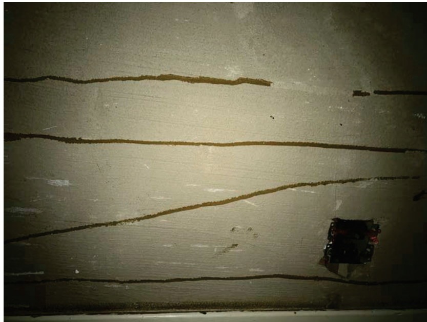
Photo 10: HA10 Tan wall glue lines on the walls of the 2 nd floor classrooms (B28-B30)
