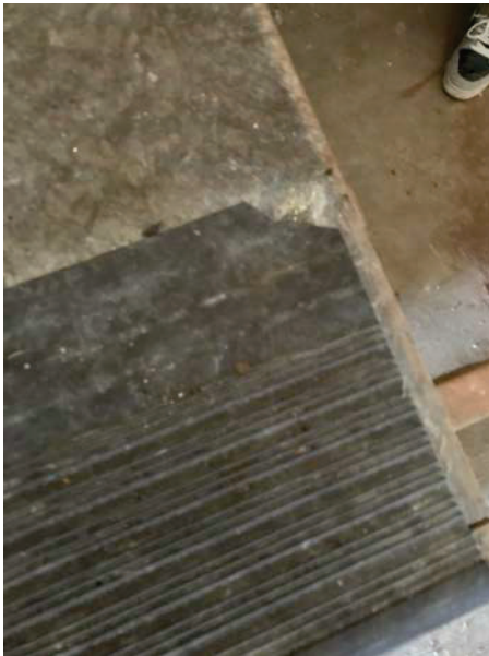
Photo 18: HA18 Brown stair covering and associated tan mastic on the stairwells of the subject property (B50-B52)
