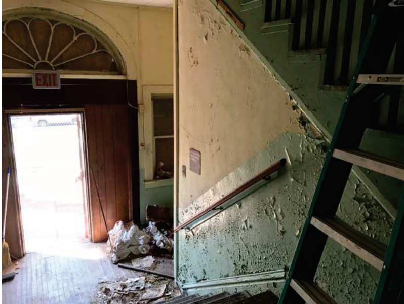
Photo 10: Entryway/Front Door [Looking towards Southwest]
