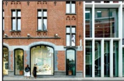
GHENT, BELGIUM REPURPOSING: REUSING BRICKS THROUGHOUT THE NEW FACADE
