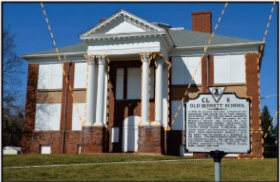
BENNETT BUILDING, MANASSAS, VIRGINIA
