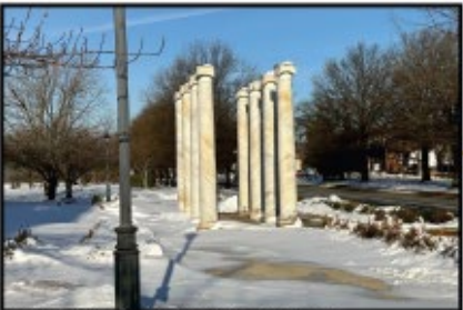
ANNE ARUNDEL COUNTY COURTHOUSE, MARYLAND CREATING SPACE: REUSE COLUMNS TO MEMORIALIZE THE STRUCTURE
