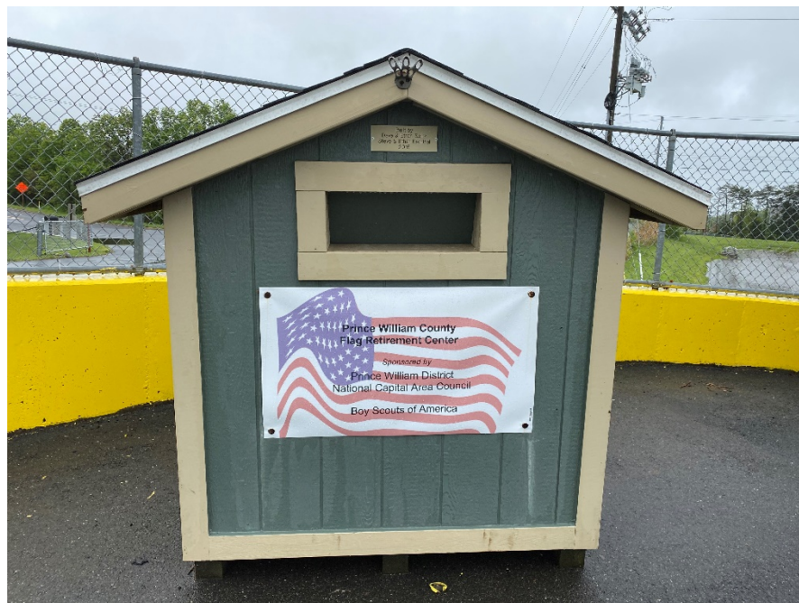
Flag collection structure at the Landfill and Balls Ford Road convenience center areas.
